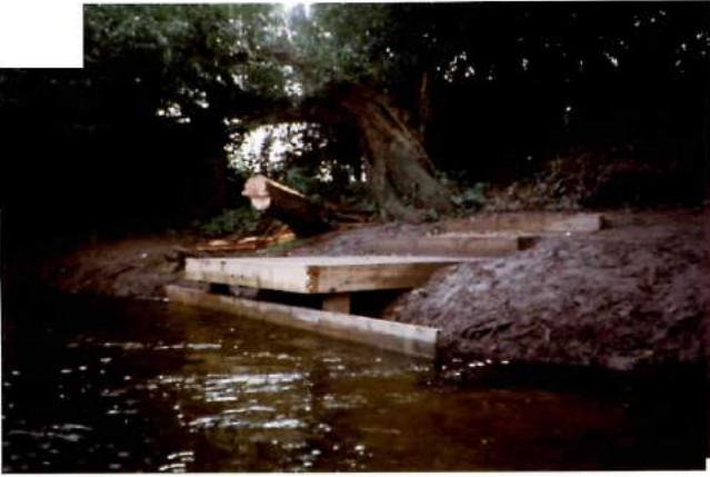
One of the canoe launching platforms installed on the Waveney in 2001 for the scheme which is now to be renegotiated to be more restrictive
