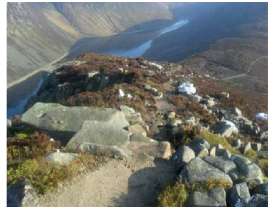
Upland Path Works on Binnian Mountain
