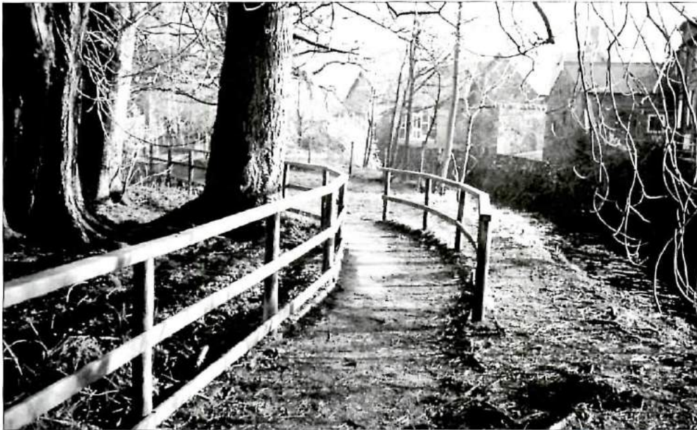
A well laid path in the Lake District National Park. A good surface, tapping rail, protection to the outside of the bend and no obstructions from overhanging branches.
