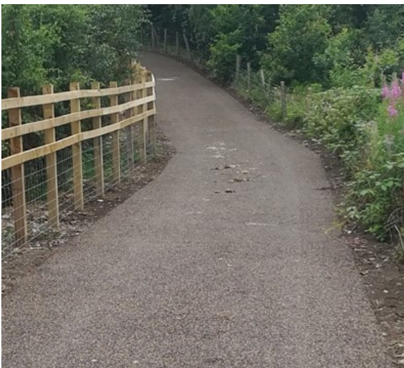
Composite rubber surfacing (Image courtesy of Sustrans)
