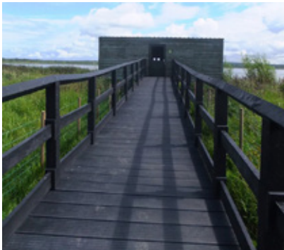
Accessible bird hide with ramped access and canopy (Image courtesy of The Wild Deck Company Ltd)
