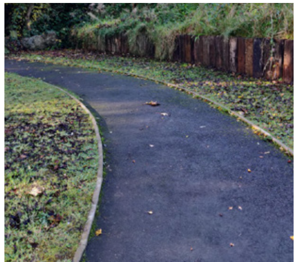
Bitmac route with defined upstand edges at start point of woodland walk
