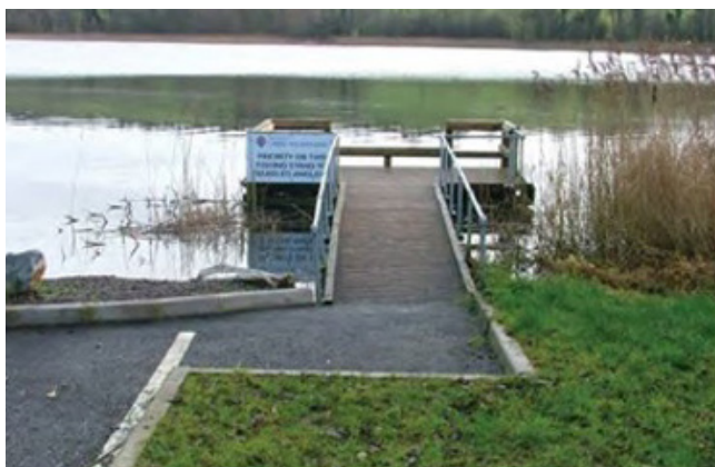
White Lough over-water fishing platform with accessible approach route (Image courtesy of Department of Agriculture, Environment and Rural Affairs)
