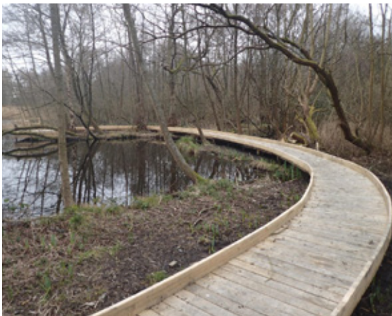
Boardwalks with edge upstands over wet ground/dipping pond (Images courtesy of The Wild Deck Company Ltd)
