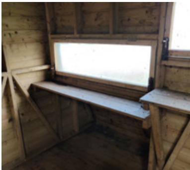
Interior showing standard viewing hatches and lowered viewing hatch with clear knee space below, shelves and rest seating at Moyola Nature Reserve
