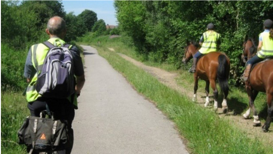
Cycle/walking lane and trotting strip with softer surface finish adjacent on shared-use external route (Image courtesy of Sustrans)
