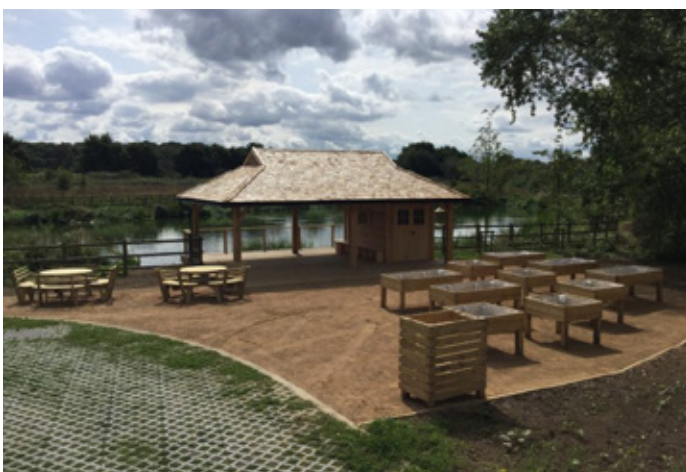
Raised planters, accessible shelter/viewing area and reinforced grass (Image courtesy of The Wild Deck Company Ltd)
