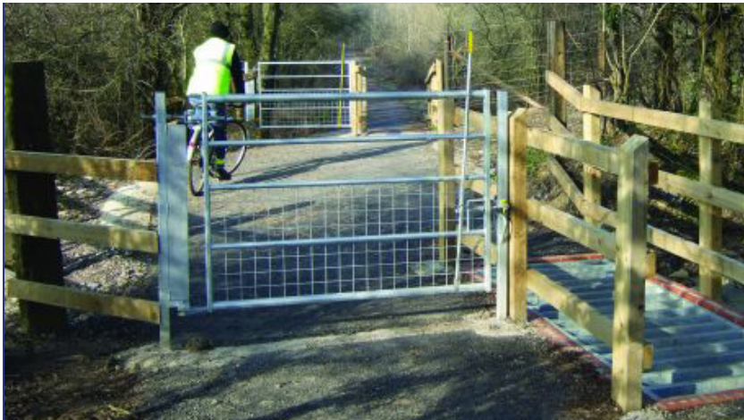
Chiltern Centrewire two-way bridle gate alongside animal grid (Image courtesy of Centrewire)
