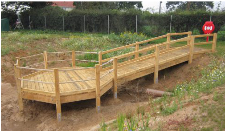
Fixed jetty/viewing platform
