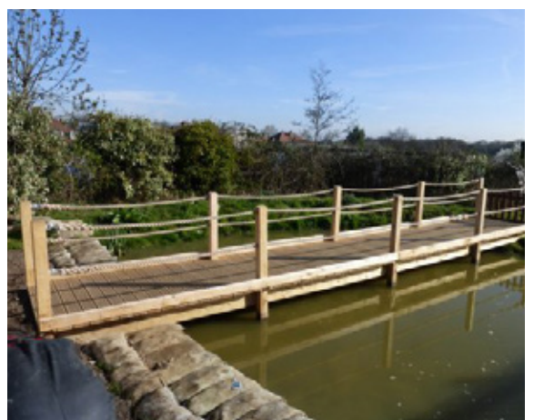
Wide bridge with edge upstands and circular profile rope handrails (Image courtesy of The Wild Deck Company Ltd)
