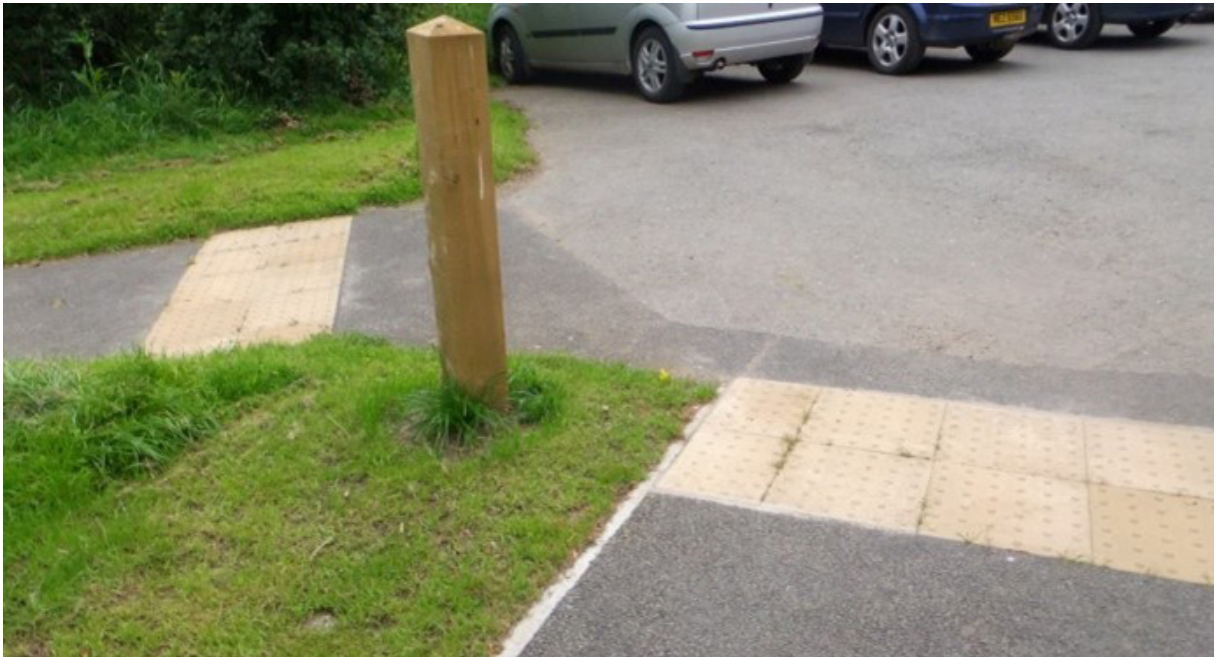
Use of tactile blister paving where external routes meet junction with car park (Image courtesy of RSPB)
