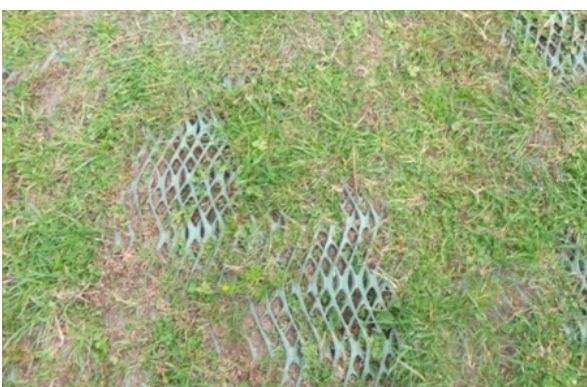
Reinforced grass surface beginning to establish
