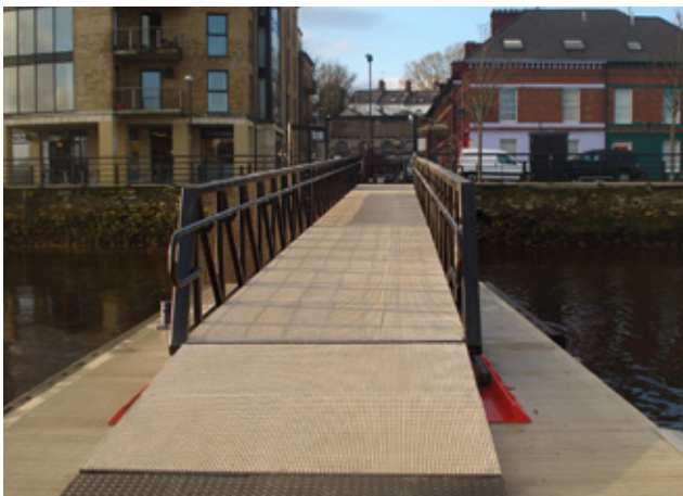
Pontoon walkway with sloping transition plate, Foyle Marina
