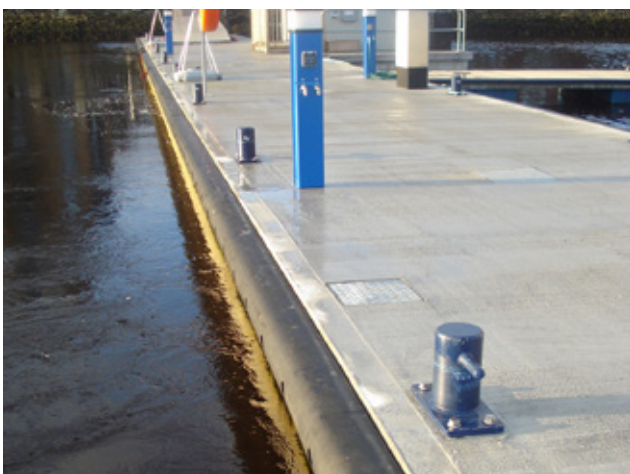
Floating pontoon, Foyle Marina
