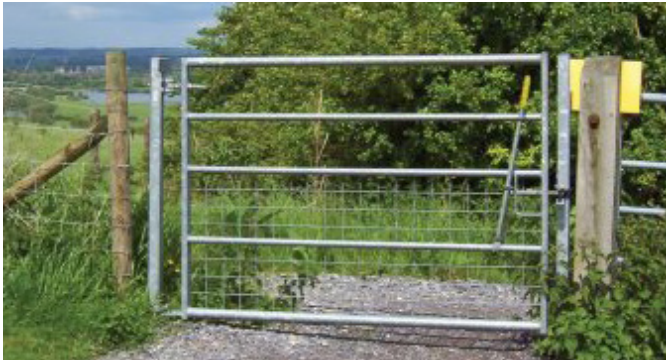
Milton Keynes Centrewire gate with contrasting latch and hardstand either side (Image courtesy of Centrewire)
