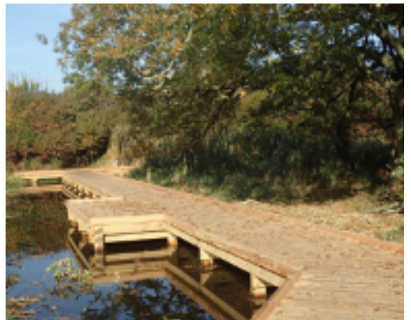
Boardwalks with edge upstands over wet ground/dipping pond (Images courtesy of The Wild Deck Company Ltd)
