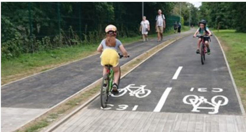
Segregation on shared-use routes and use of tactile paving (Images courtesy of Sustrans)
