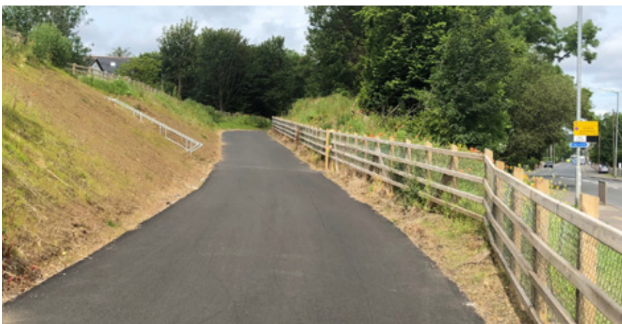
Comber Greenway – bitmac surface and roadside protective fencing (Image courtesy of IMTAC)
