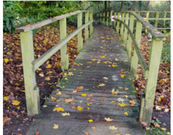
Bridge over uneven ground, with gently sloped transition area
