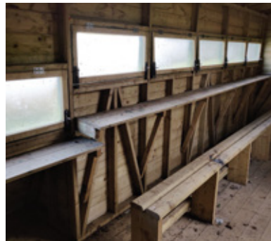
Interior showing standard viewing hatches and lowered viewing hatch with clear knee space below, shelves and rest seating at Moyola Nature Reserve
