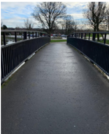
Firm bitmac surface on access bridge, Victoria Park Belfast
