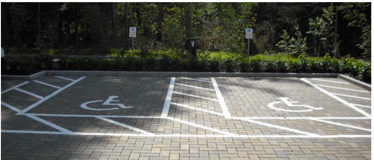
Formal accessible parking area
